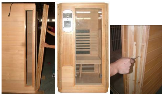
FIG-9 Install front panel
