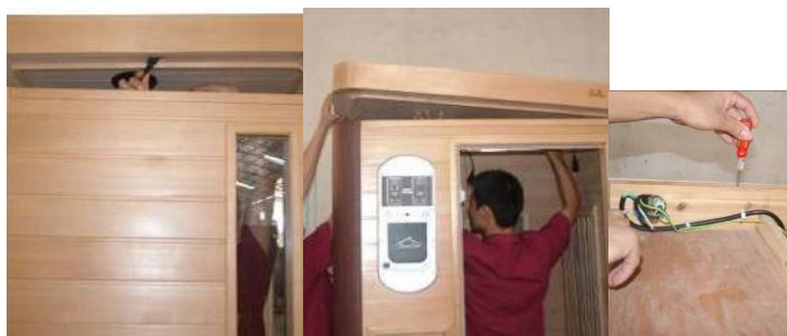
FIG-10 Install top panel
